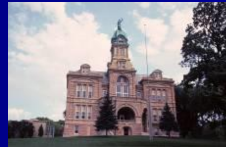
Blue Earth County Courthouse Mankato, MN
