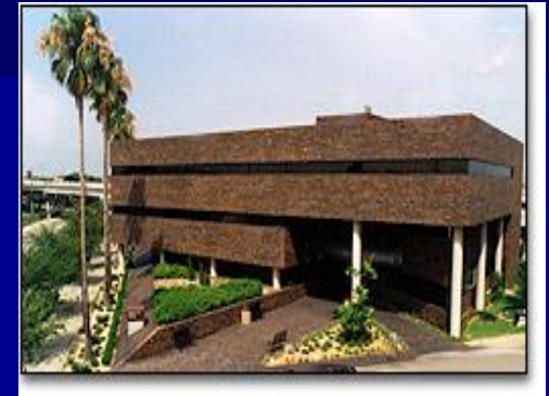
Hillsborough County Water Department Administration Building Hillsborough County, FL
