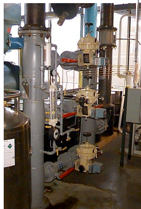
Figure 3: Primary Regulator Valves
