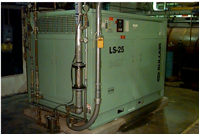
Figure 2: High Efficiency Enclosed Compressor
