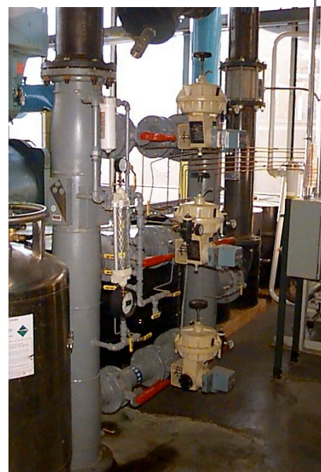
Figure 3: Primary Regulator Valves
