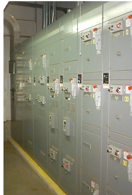
Figure 4: Variable Frequency Drives
