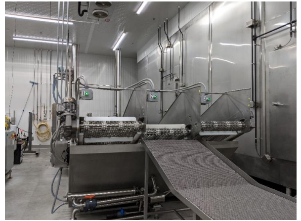
Conveyor off of three lane chiller
