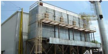
Baghouse for Control of Particulate Emissions from Wood-Fired Boiler
